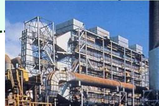
Cleaner Production and pollution control equipment
